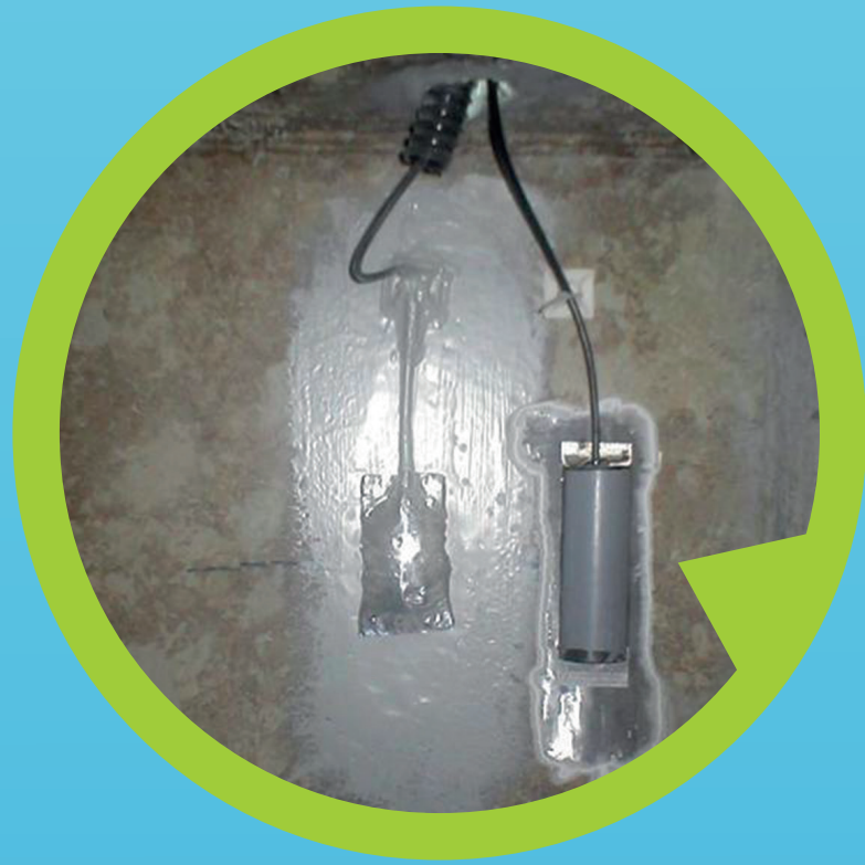
water dam (Gabčíkovo) flooded with water
